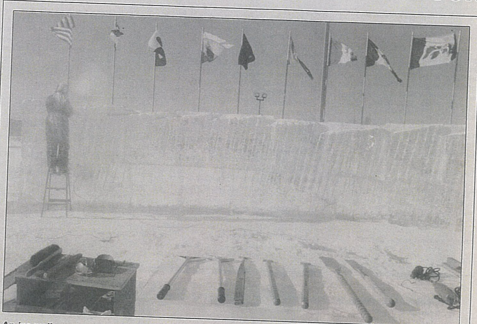
An ice wall was constructed in Town Square last week to be used as a backdrop for various awards ceremonies. Ice for the wall was brought down from quarries in Fairbanks.
